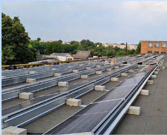
Ballasted mounting in Hungary
