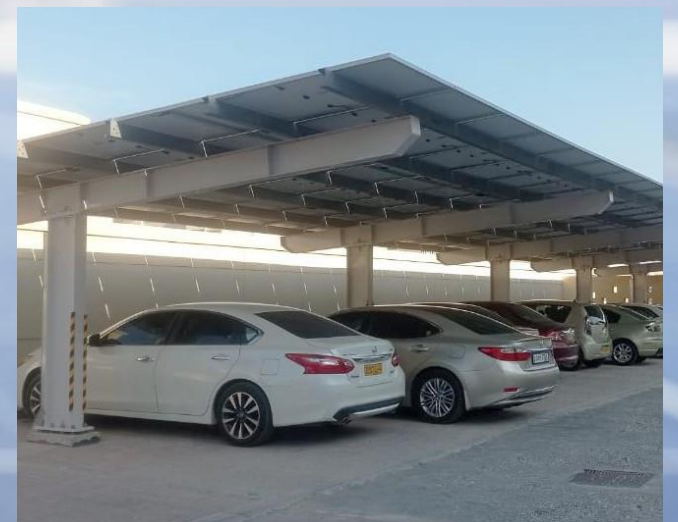
Steel solar carport in Oman
