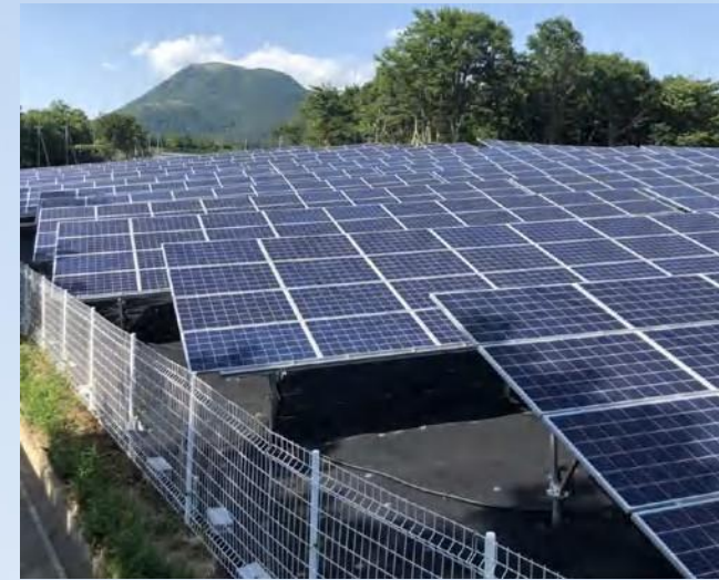
Aluminum ground mounting in Japan
