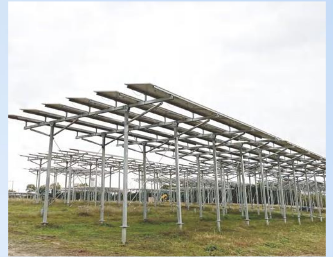
Steel ground mounting in Japan
