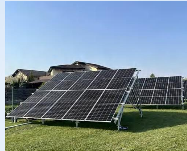
Aluminum ground mounting in Austria
